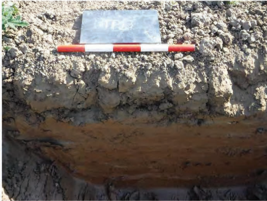
Plate 5 TP13, looking north-east
